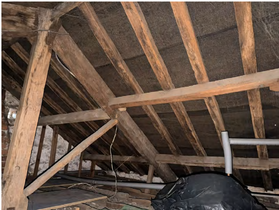
ROOF VOID SHOWING BITUMEN UNDERFELT
