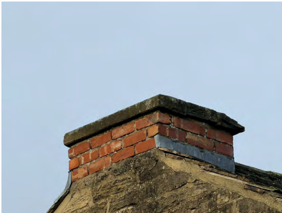
REDUCED CHIMNEY STACK
