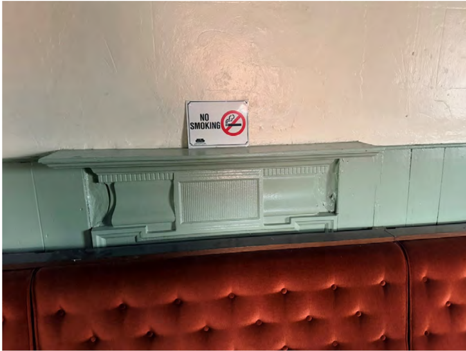
FIREPLACE TO WEST WALL (CONCEALED BEHIND SEATING)
