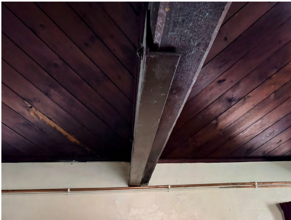
STEEL REPAIR TO ROOF TRUSS
