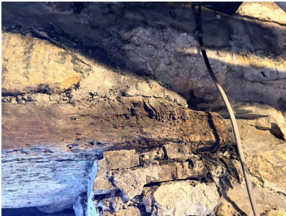
TIMBER LINTEL OVER WEST ELEVATION DOOR
