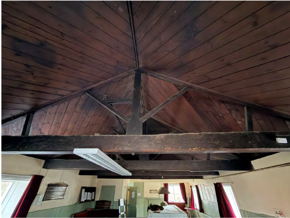
ROOF TRUSSES AND SLOPING CEILING IN SNOOKER ROOM
