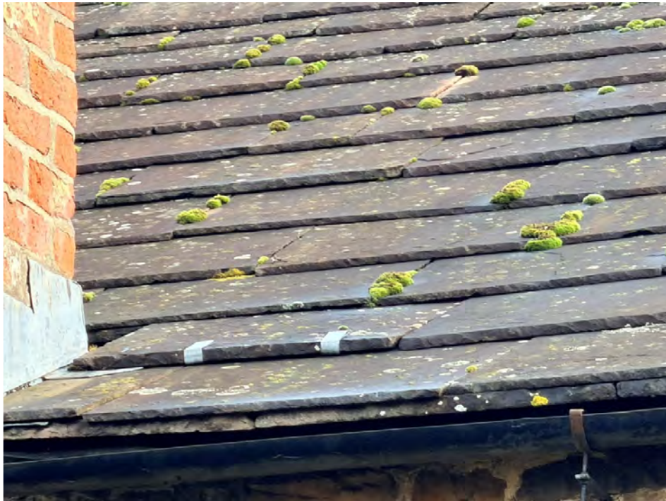
CLIPPED SLATE AND MOSS TO WEST ROOF SLOPE
