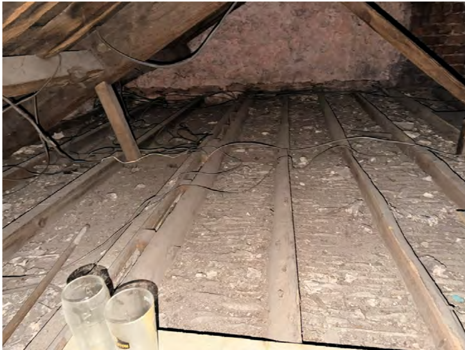
UPPER SIDE OF LATH & PLASTER CEILING OVER SNOOKER ROOM
