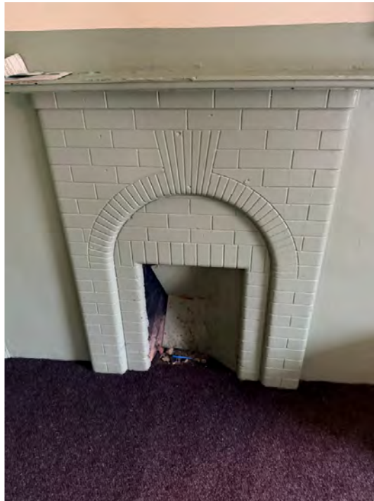
REDUNDANT FIREPLACE ON SOUTH WALL AT FIRST FLOOR
