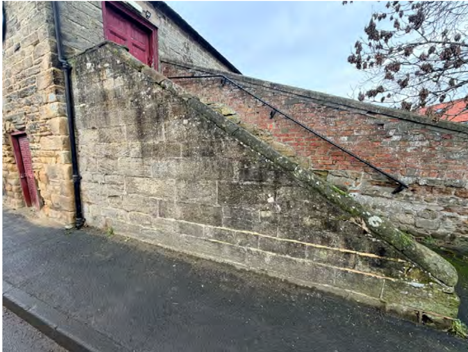
SOUTH WALL TO EXTERNAL STAIRCASE
