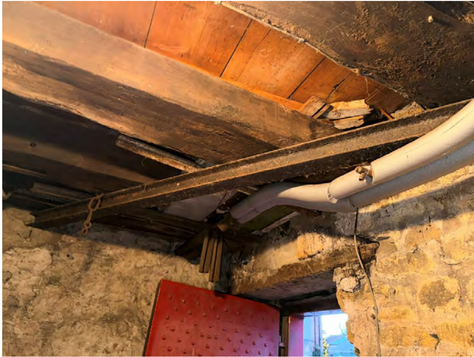
HSITORIC REPAIR AND STEEL SUPPORT TO FIRST FLOOR JOISTS
