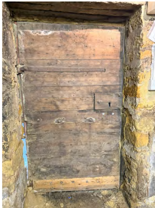
REVERSE SIDE OF DOOR TO SOUTH ELEVATION
