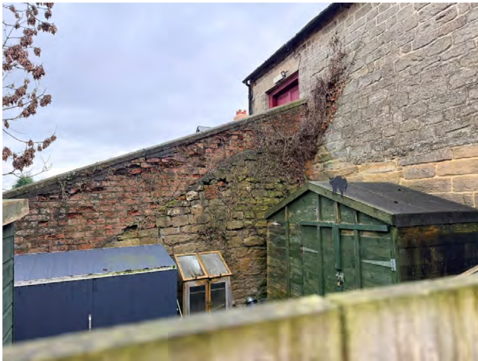
NORTH WALL TO THE EXTERNAL STAIRCASE
