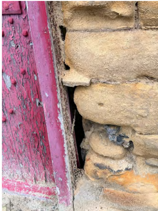
BASE OF DOOR AND FRAME TO SOUTH ELEVATION
