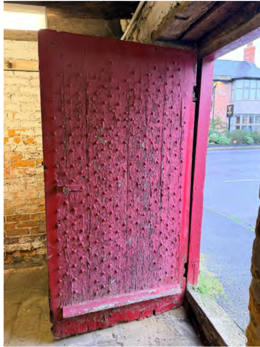
WEST ELEVATION DOOR
