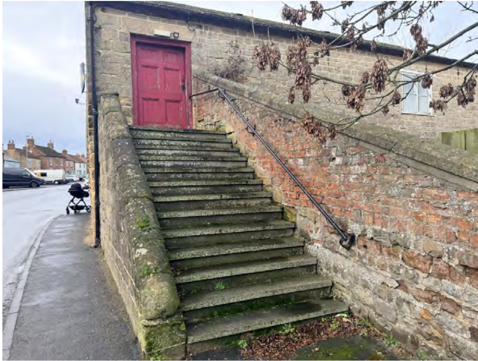
EXTERNAL STAIRCASE TO EAST ELEVATION
