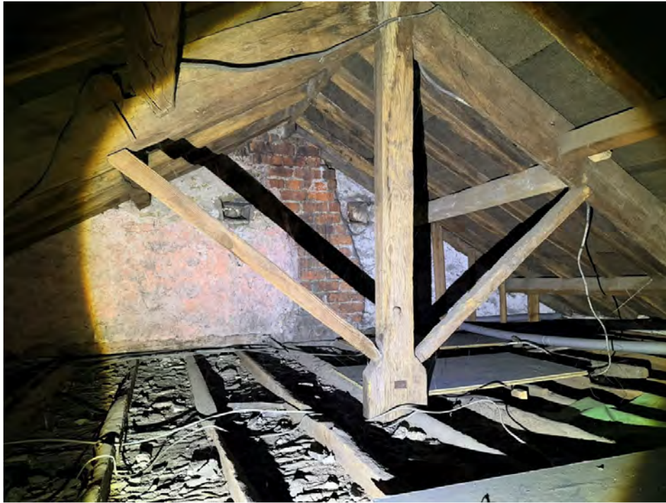
ROOF SPACE OVER SNOOKER ROOM
